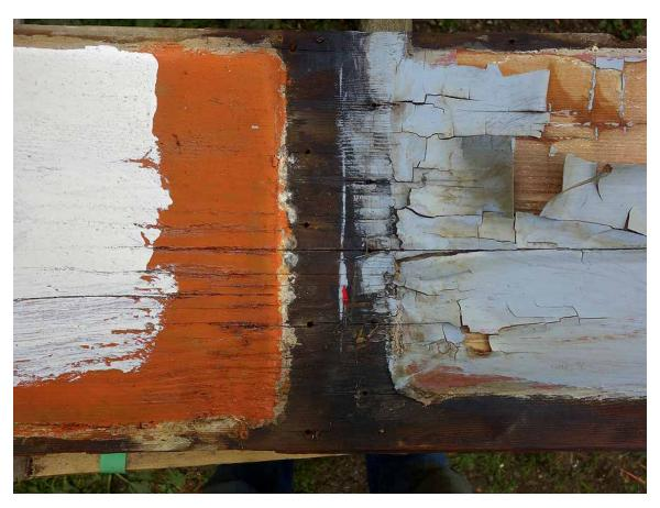
Ceiling—Removed twelve-inch-wide ceiling board shows various layers of paint.
