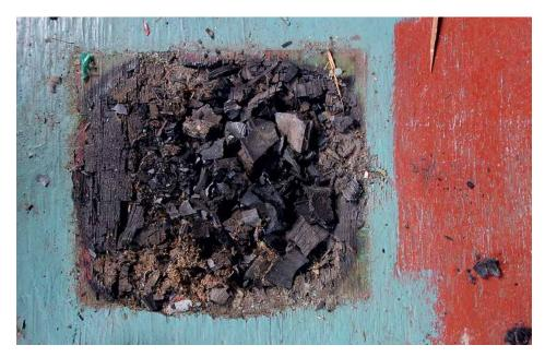
It Almost Burned Down—Consecutive images show burn area filled with cinders then cleared to reveal the damage through almost three inches of floor.
