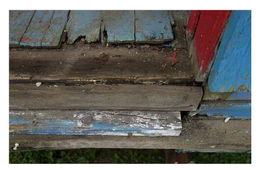
Threshold—Disintegration of the doorway evident after removing the sill.
